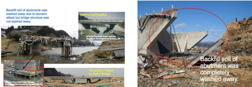
Figure 1: Bridge Damages during Earthquake and Tsunami (CAESAR, 2011)
